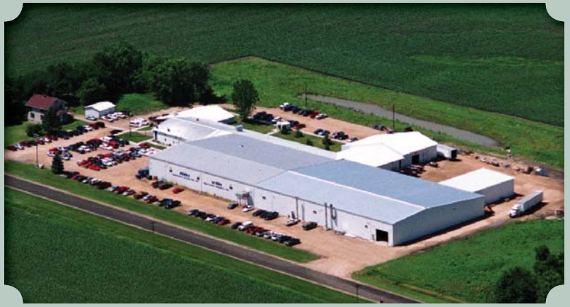
MEI Manufacturing Headquarters | Mankato, MN
